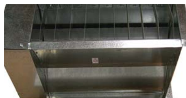
Diffuser back with straightening vanes
